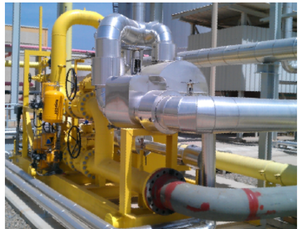
Gas turbine plant and gas fuel pre-heating system.
